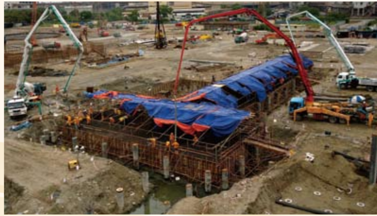
马来西亚Prai CCGT电厂土建施工项目 Onshore Civil Work Project of Malaysia Prai CCGT Power Plant
