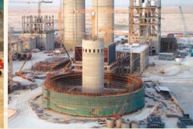
仓体滑模 Slip form of bin
