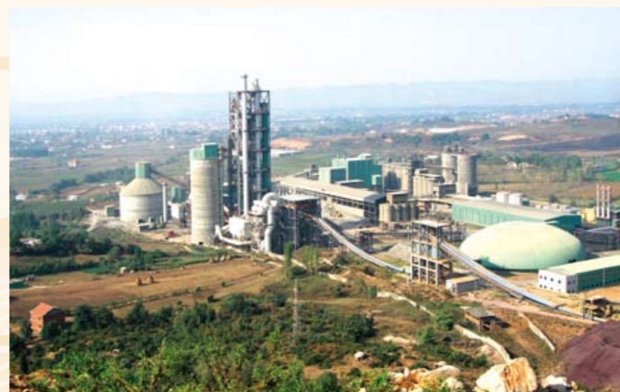
阿尔巴尼亚FUSHE KRUIJE水泥厂 (3300 t/d) Albania FUSHE KRUIJE cement plant (3300 t/d)
