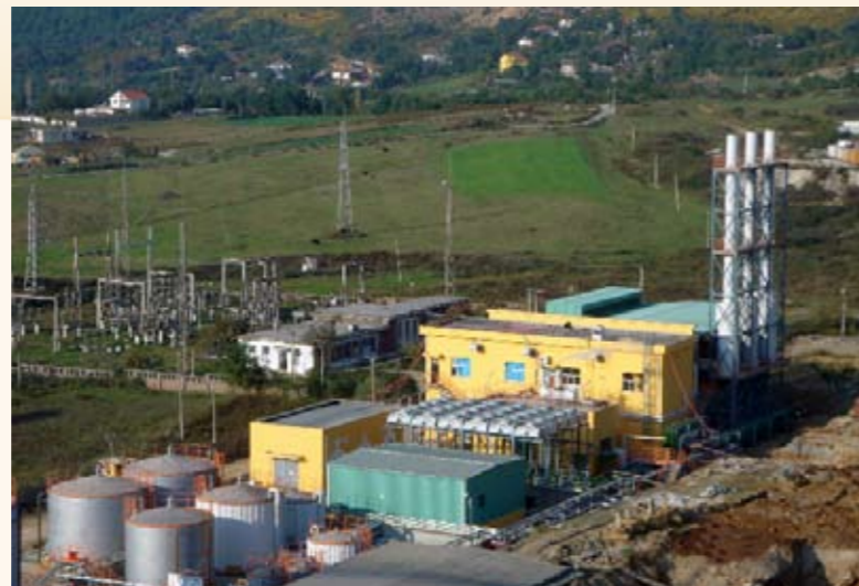
阿尔巴尼亚FUSHE-KRUJE重油发电厂 Albania FUSHE-KRUJE Heavy Oil Power Plant
