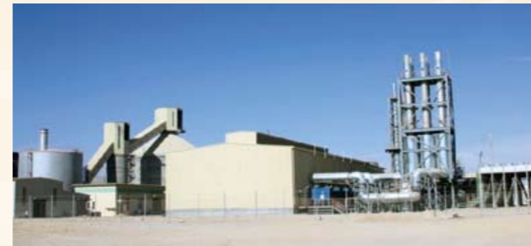
叙利亚ABC重油发电厂 Syria ABC Heavy Oil Power Plant
