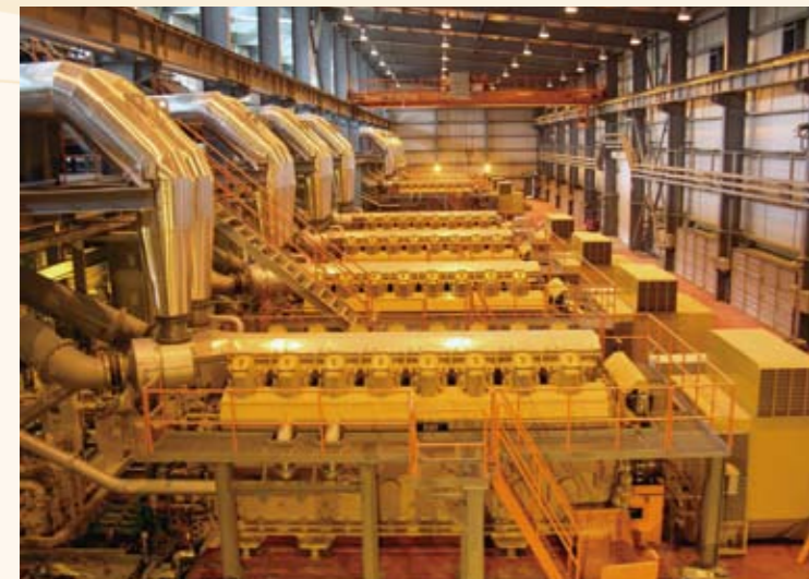
沙特SPCC重油发电厂 Saudi Arabia SPCC Heavy Oil Power Plant
